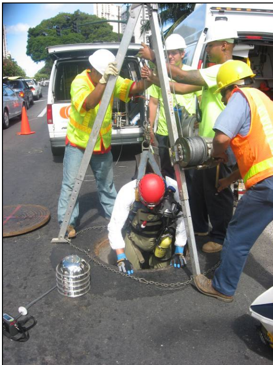
Photo 3.1 – Confined Space Entry
