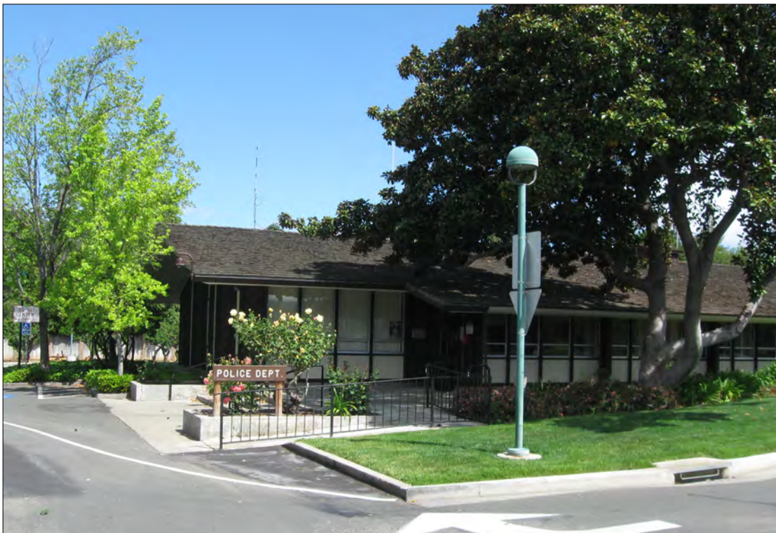
Photo 8 - View of the existing Police Station. This building would be demolished and a parking lot serving the new Community Center would be constructed at this location under the proposed Master Plan. The magnolia tree shown on the right side of the photo would be removed.
