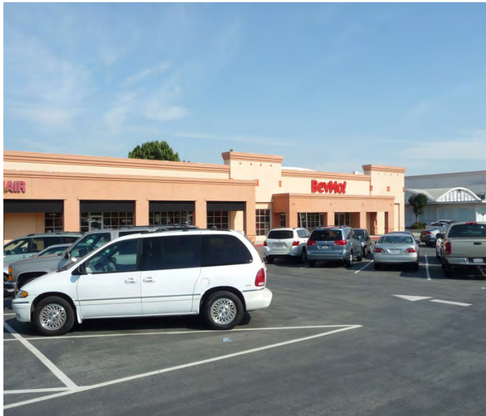
Photo 4: Kumon, Math, Reading Success north side store front, Machado Commercial Building
