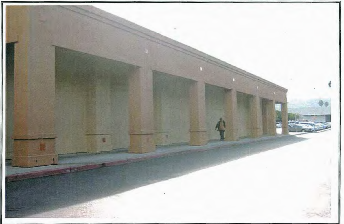
Photograph Number 2 North perimeter of building
