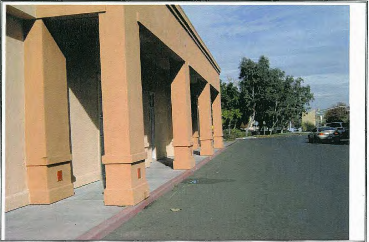
Photograph Number 4 South side of building, driveway
