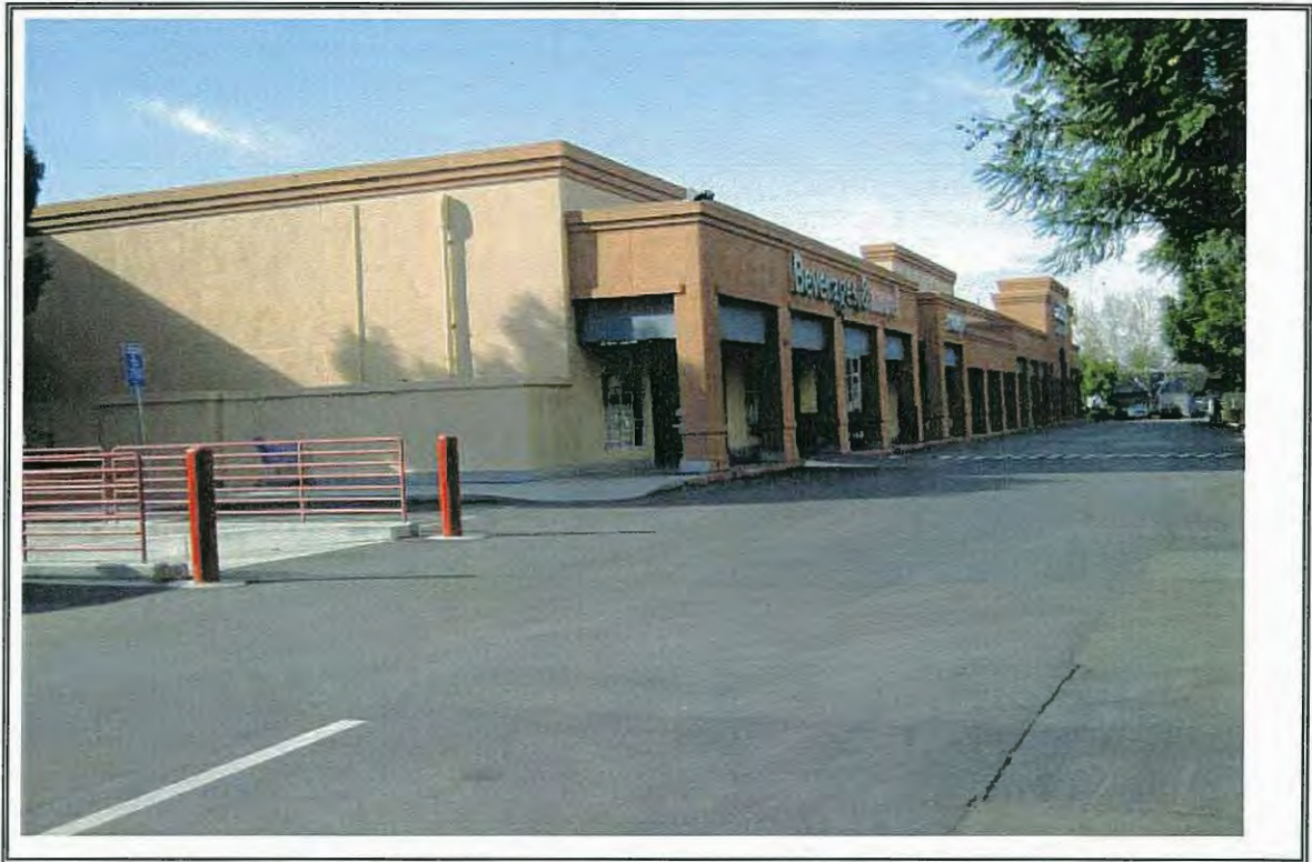
Photograph Number 3: East side of building
