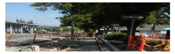
The annual concrete sidewalk and curb/gutter repair project is intended to address the highest priority repair locations. The primary focus is on the replacement of damaged sidewalks that represent hazards to pedestrians. Staff continually receive complaints from residents regarding cracks or uplifted sidewalks that could cause a "trip and fall" type accident. This project provides for replacement of cracked or uplifted sidewalks throughout the City that cannot be patched or ground down.
