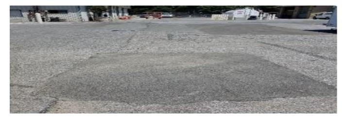
The pavement at the City's Municipal Services Center (MSC) is deteriorating and in need of repair. This project will include the design and construction of pavement rehabilitation and improvement of the current drainage system. The design will also incorporate the green infrastructure features into the project to comply with the current stormwater permit requirements.
